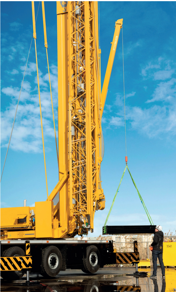
Auxiliary crane for placing the steel pads
