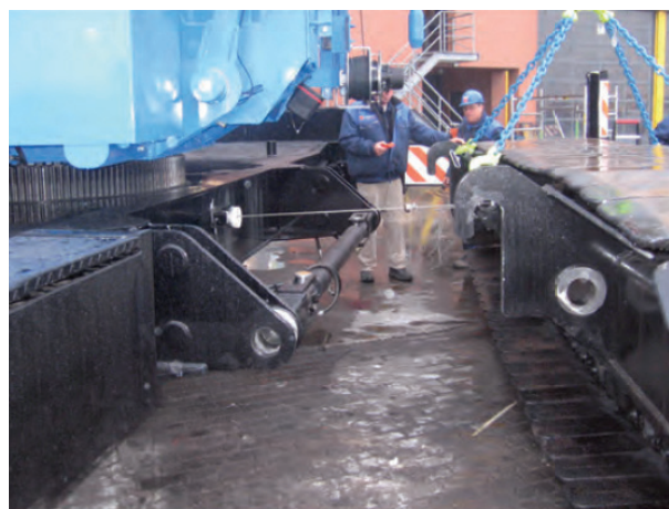
Manoeuvre track towards chassis
