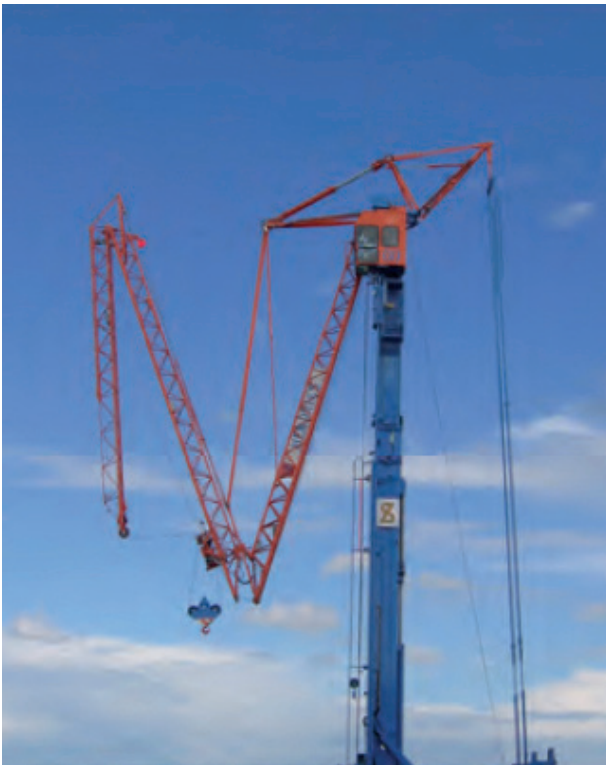
Erect the crane
